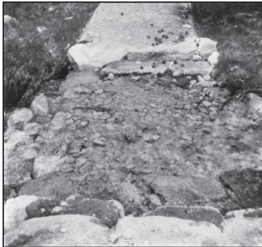
Figure 28—Wide cross drain and causeway.
