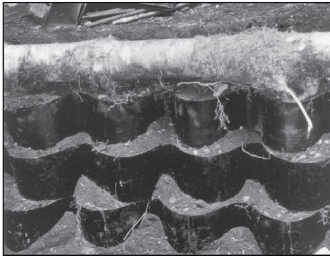
Figure 39—"Flower pot" retaining wall of geocells.
