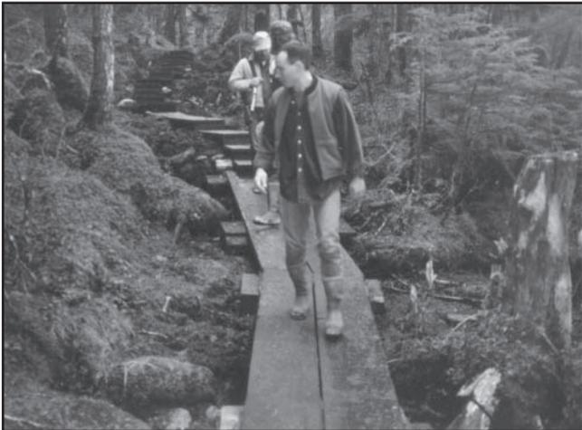
Figure 65—Step and run stairs in Alaska (plank boardwalk in foreground).
