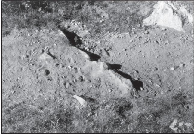
Figure 21—Waterbars need to be constructed at a 45 to 60° angle to the trail. Water should run off the trail before hitting the waterbar.
