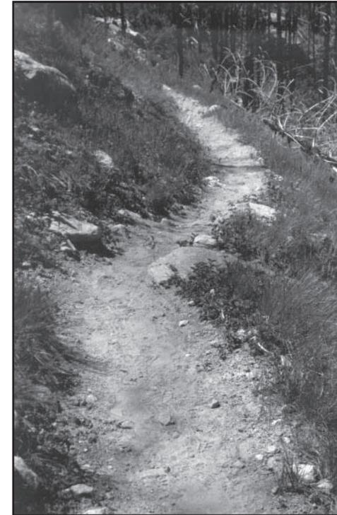
Figure 7—Rocks and logs help to keep the trail in place. And remember that this is a path through nature, not a monument to Attila the Hun.
